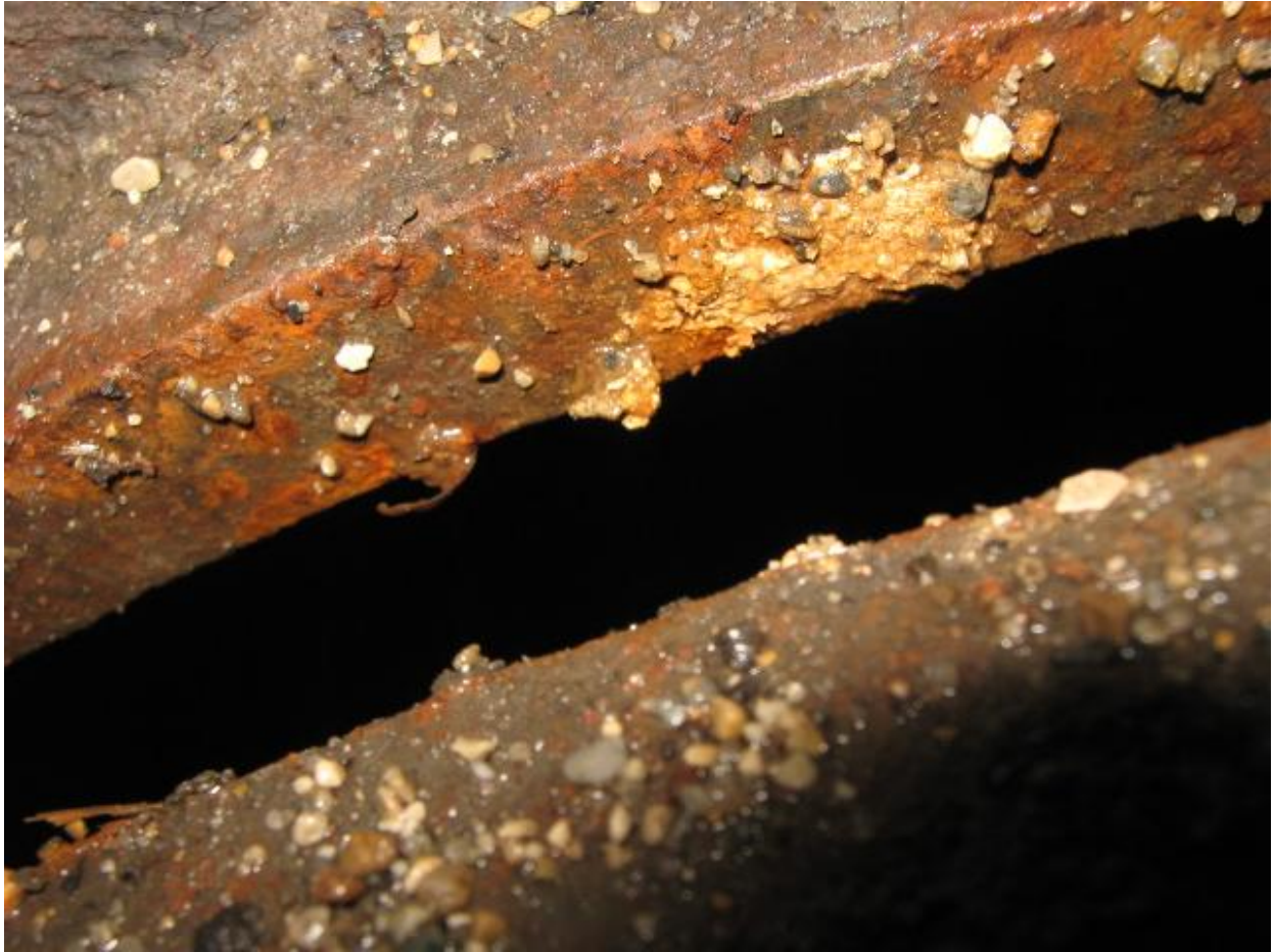
Figure 3 – Small debris stuck on gate frame seating face
