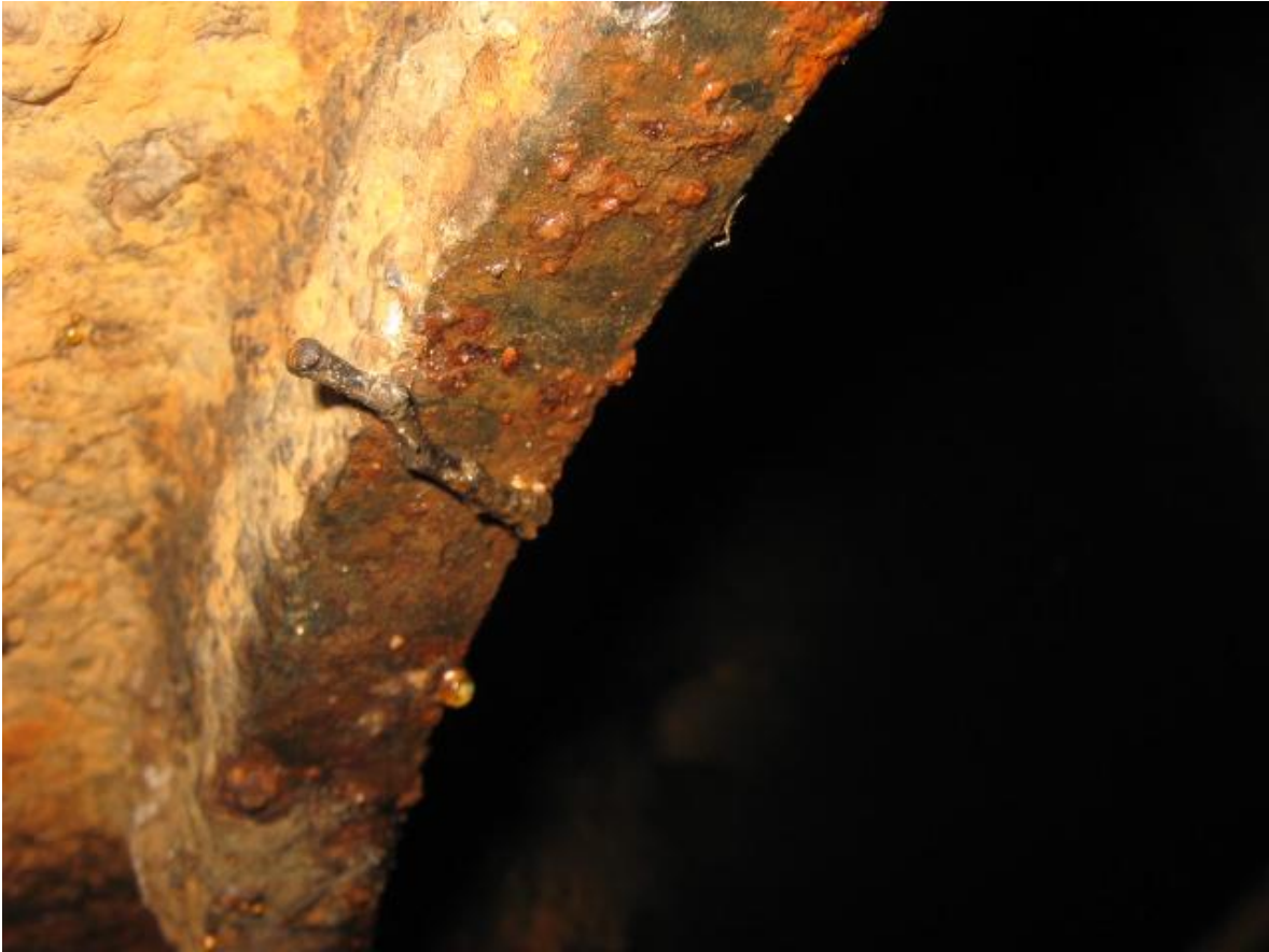
Figure 4 – Small stick stuck to corrosion on gate frame seating face
