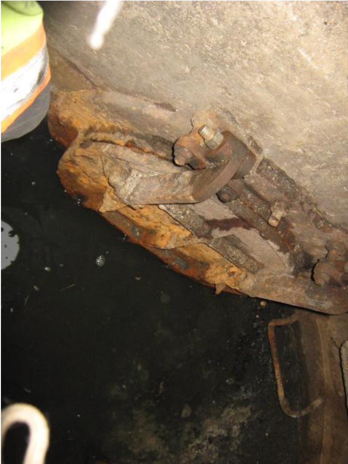
January 28, 2015 Inspection of Flap Gate near Sturgeon Creek at Ness Inspection by Kyle Sanders, Service Technician, Power & Mine Supply Service Group
