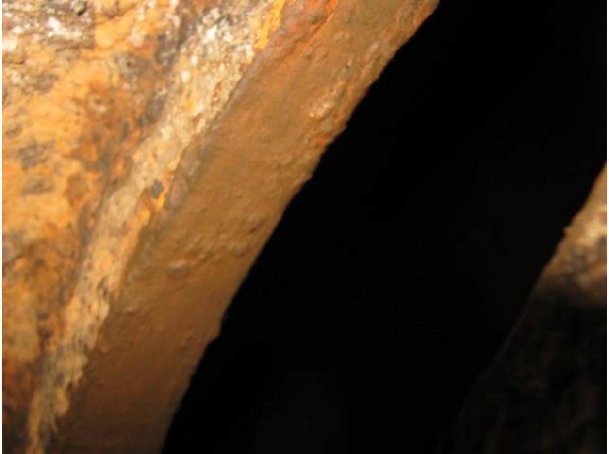
Figure 6 – Gate frame seating face after being wiped down with a work glove
