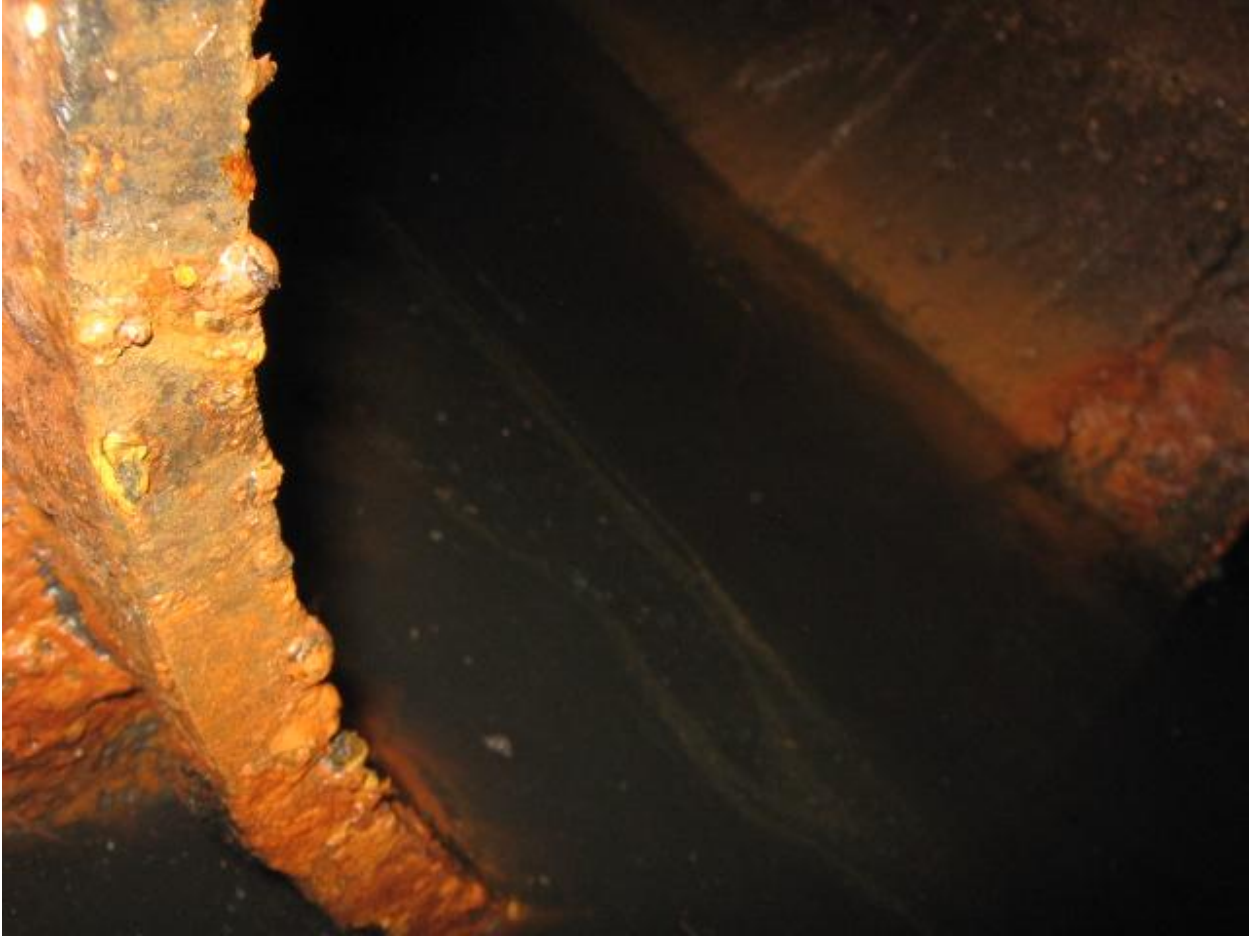
Figure 2 – seating face of gate frame
