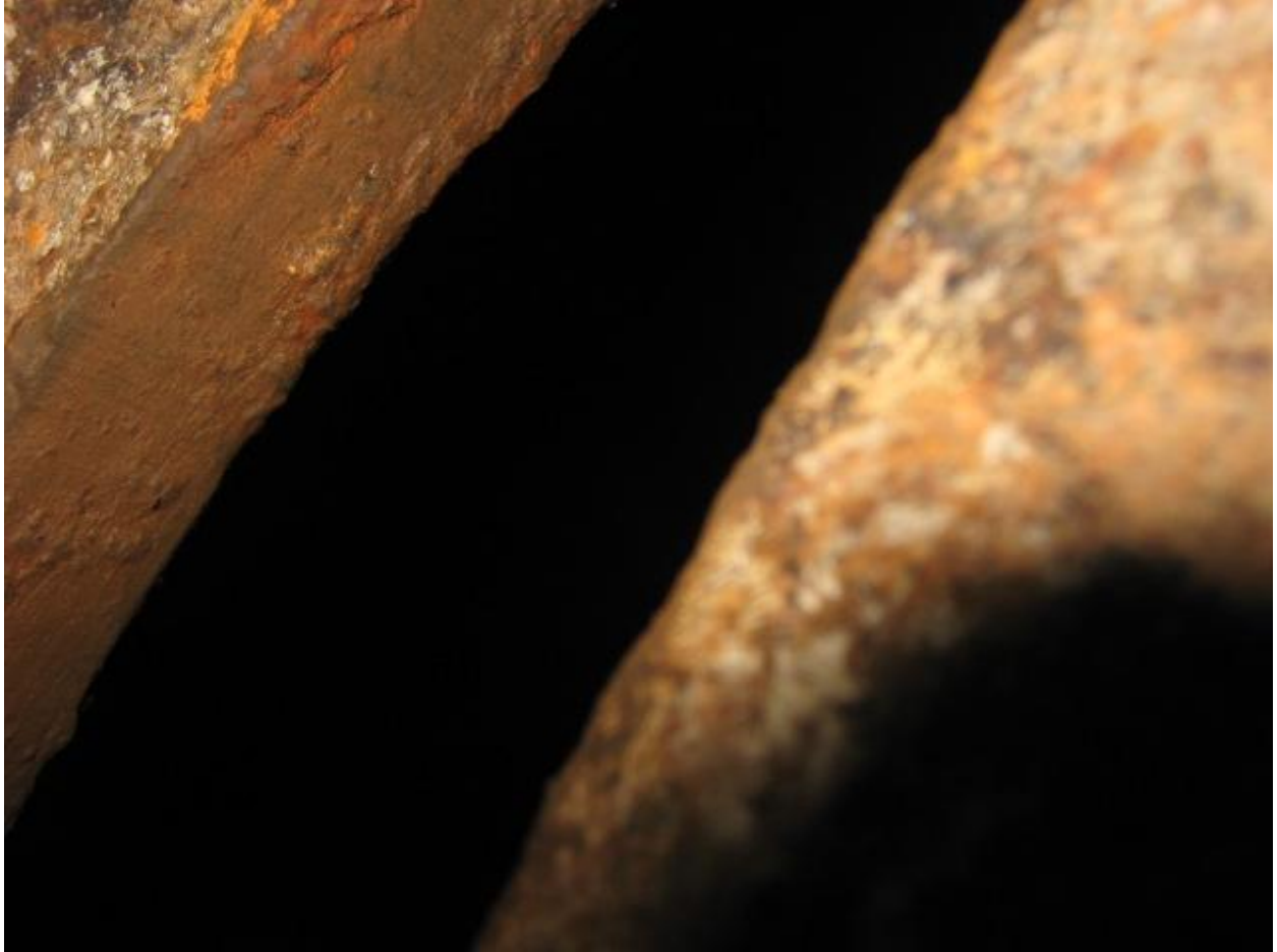
Figure 5 – Gate frame seating face after being wiped down with a work glove
